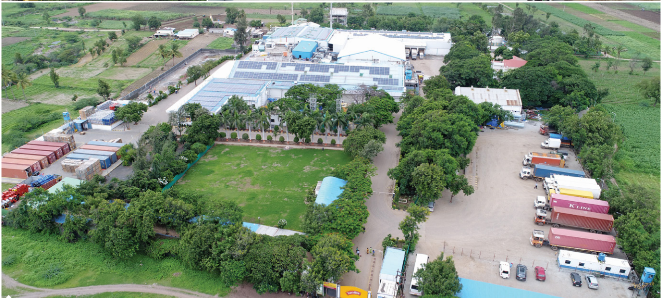
Roof top Solar Plant
